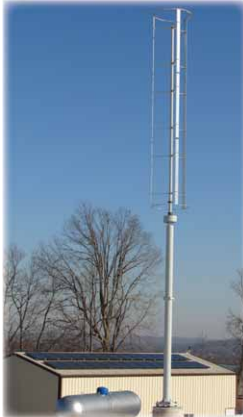
Hanschen's wind spire is four feet wide by 20 feet high, has four blades and spins like a circle. The capacity with an eight-mile an hour wind is 1.2 kW (1,200 watts). The installed cost of the wind spire in November 2009 was approximately $11,000.
